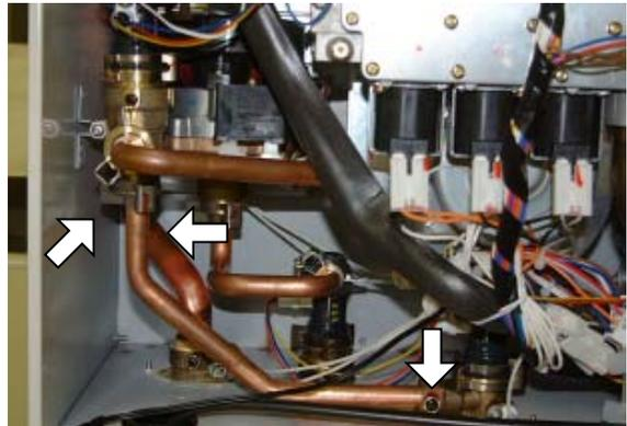
(2) Remove the quick fastener of the water flow sensor set 1 and the discharge hot-water pipe locking screw.
