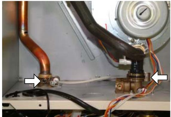
(3) Remove the connecting quick fasteners of the water flow sensor set 3 adjustment valve and the water flow servo set 2, and the mixing body block locking screw.
