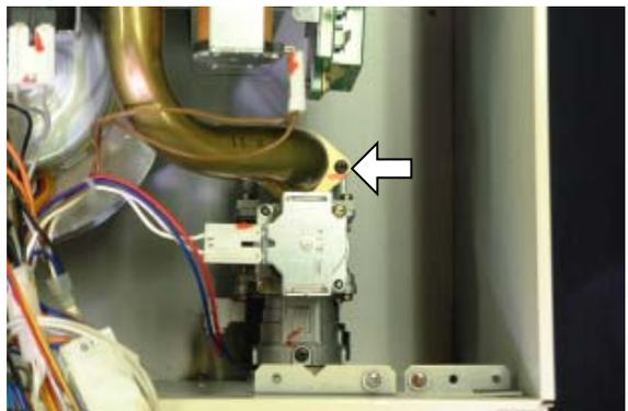
(2) Remove the fasten terminal of the gas electromagnetic valve, then remove the 4 manifold locking screws.
