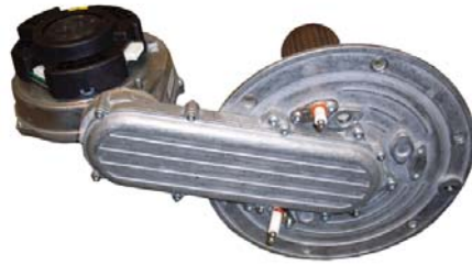
Removed Burner Assembly
